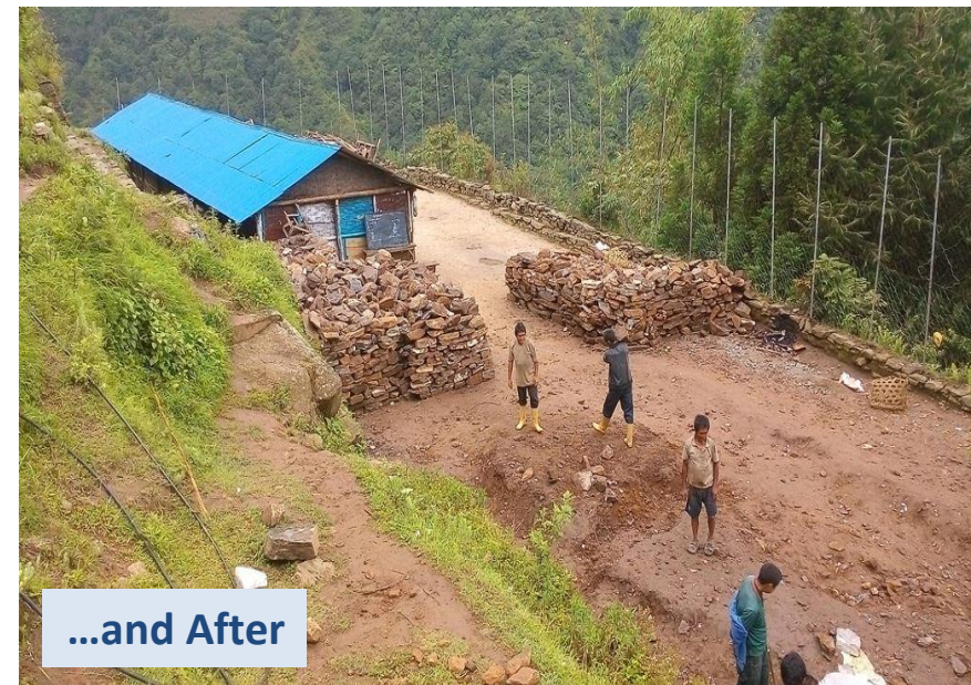
Community clearing terrace by hand in Lungthung, Taplejung
